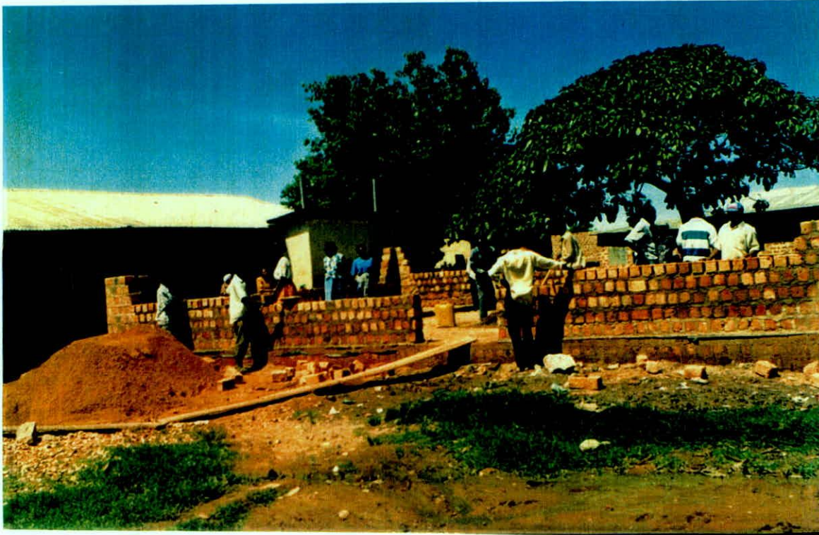
Construction site with staff in the background
